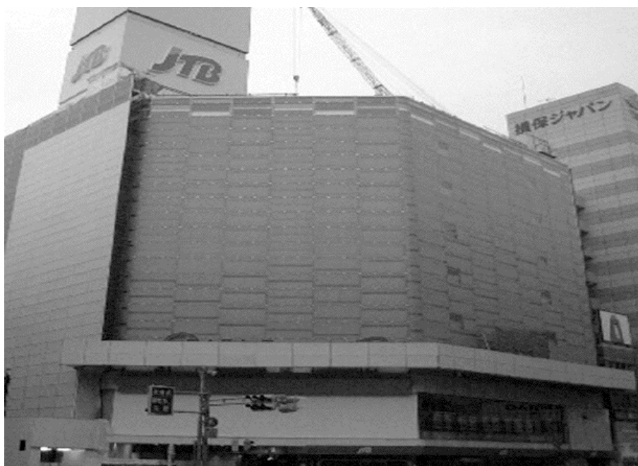
Fig. 5 Outlook of EB film applied fro building outside wall surface.
