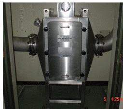
1st Stage Charcoal Filter Housing Installation Completed
