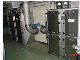
2nd Stage Charcoal Filter Housing Installation Completed
