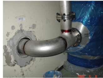
Duct Welding & Liquid Penetration Test
