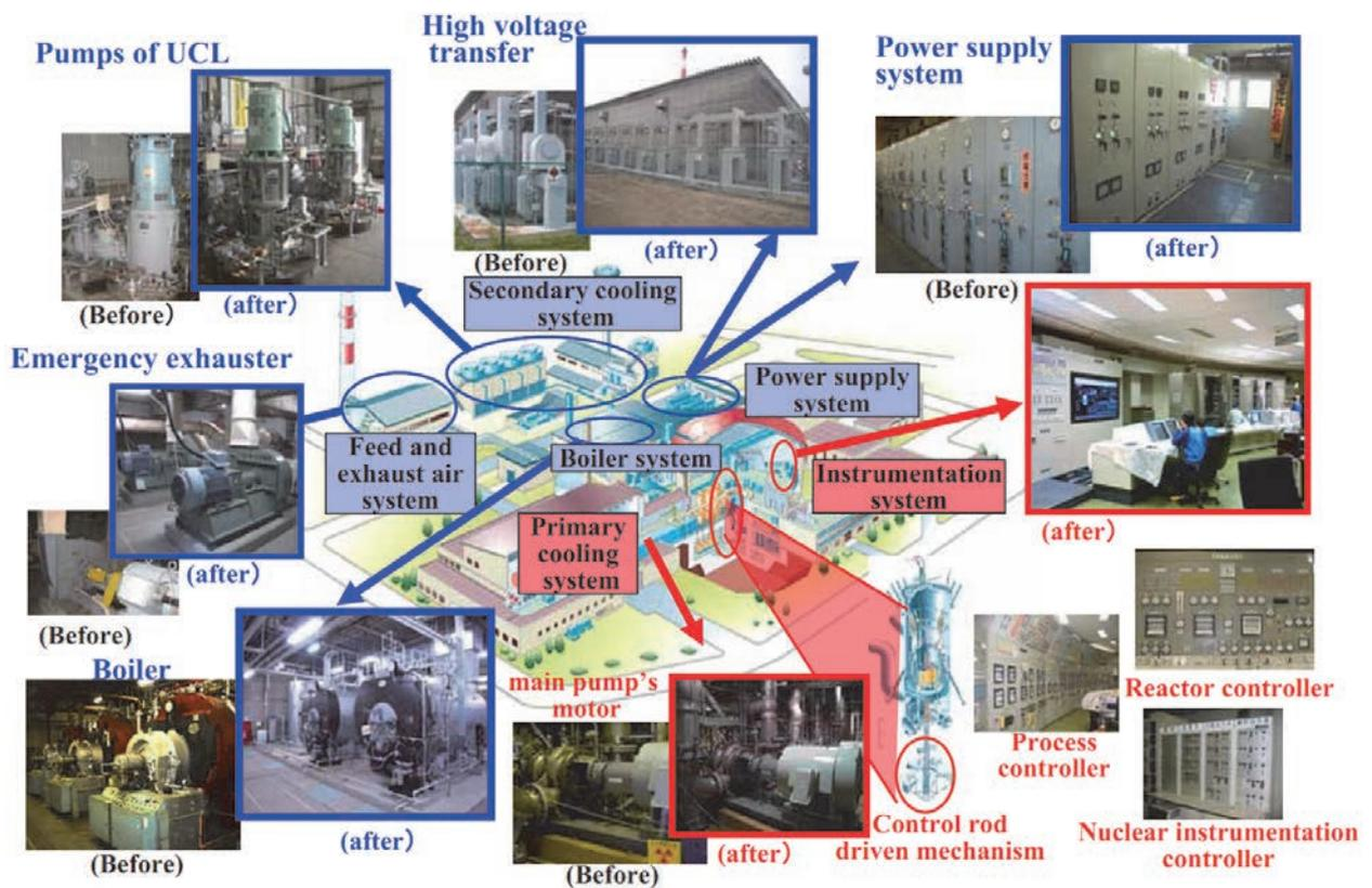
Fig.2 Outline of the refurbishment of reactor facilities
