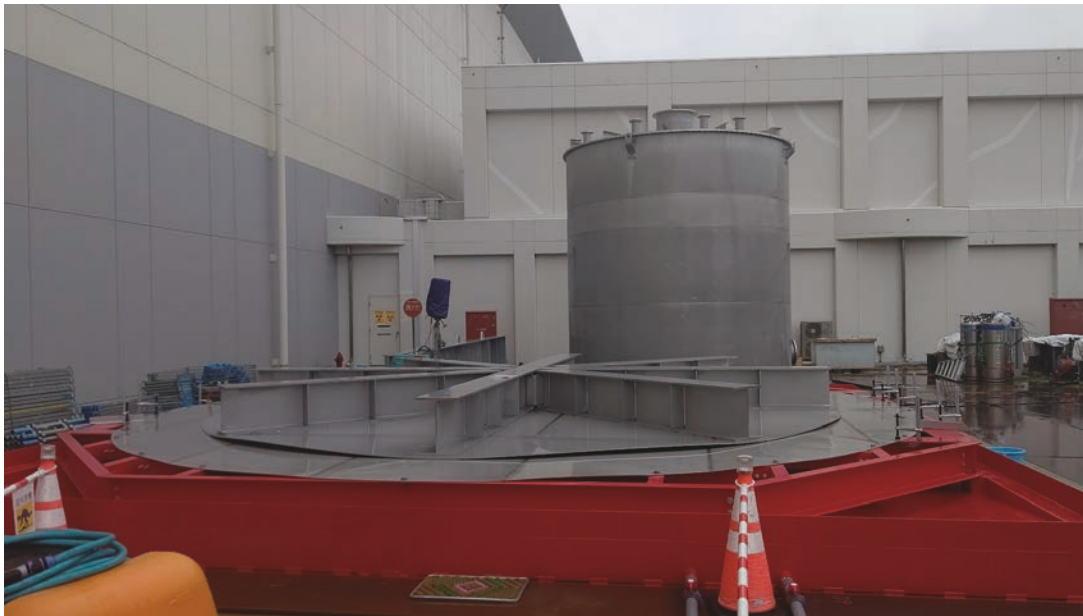
Figure 3: The status of s.s. tank construction of the JSNS 2 -II as of 17 December 2021. The inner s.s. tank can be seen in the back, while the base of the detector and the support structure of the outer s.s. tank can be seen in the front.
