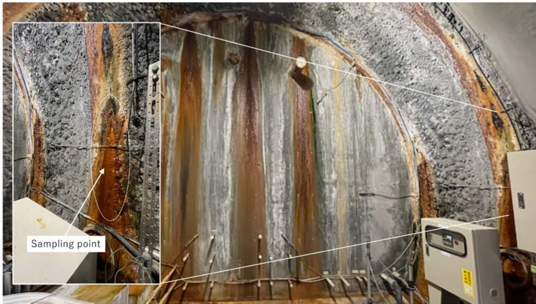
Fig. 2 Picture of sampling point of the EBS-leakage water
