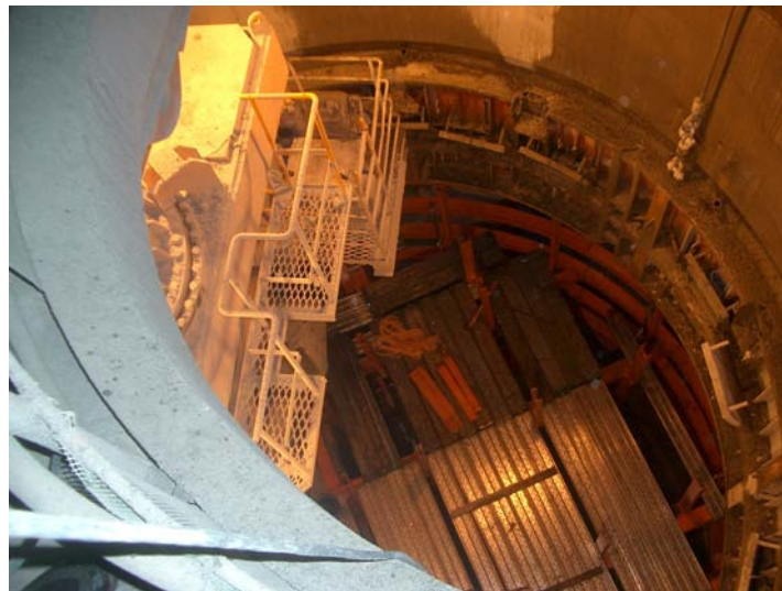
Figure 1.4: Inside the Ventilation Shaft, looking down to the shaft bottom
