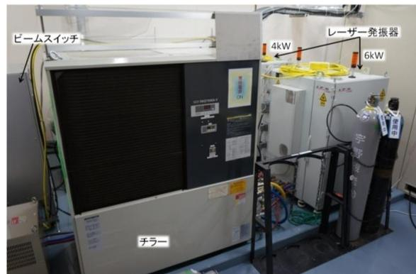
Fig. 5 Laser oscillator and water-cooled chiller of 10 (6+4) kW fiber laser
