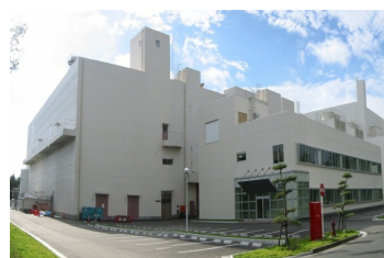
② Volume Reduction Facilities
