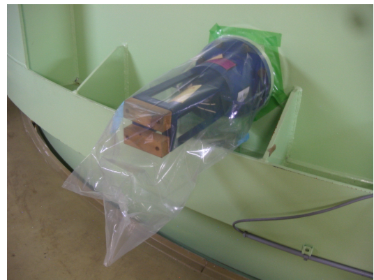
Fig. 3. Collecting leaking SF 6 gas in a plastic bag for searching leak spots.
