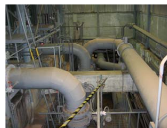
Secondary cooling system pipes 450A
