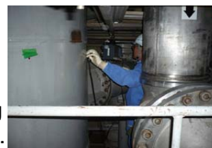
Thickness measurement by the ultrasonic thickness gauge
