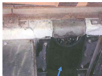
Canal expansion joint
