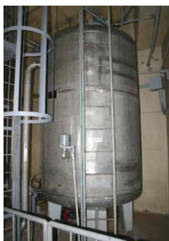
Purify water tank 3160 mm H x 1486 mm \phi
