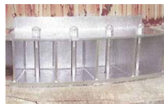
After repairing and paints
