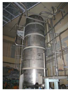
Degas tank 6200 mm H x 1566 mm \phi
