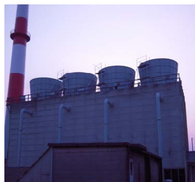
JMTR secondary cooling system cooling tower (4 cells)
