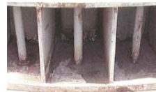
Removing paints and rusts from the investigation part
