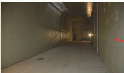
A view into basement area of Linac tunnel for LEHIPA facility
