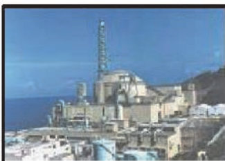
Prototype FBR, MONJU 280 MWe/Three-loop Started testing with zero-power in 2010
