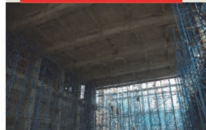
High-bay area above LEHIPA linac tunnel in basement
