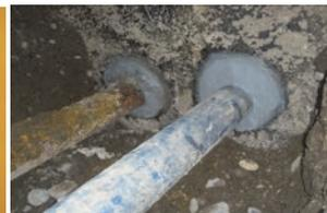
Photo. 3 Repair of the penetration part of a subterranean wall.
