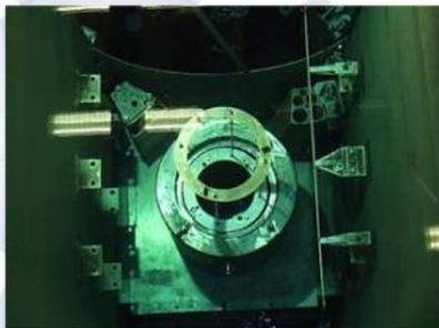
Installing the lifting yoke
