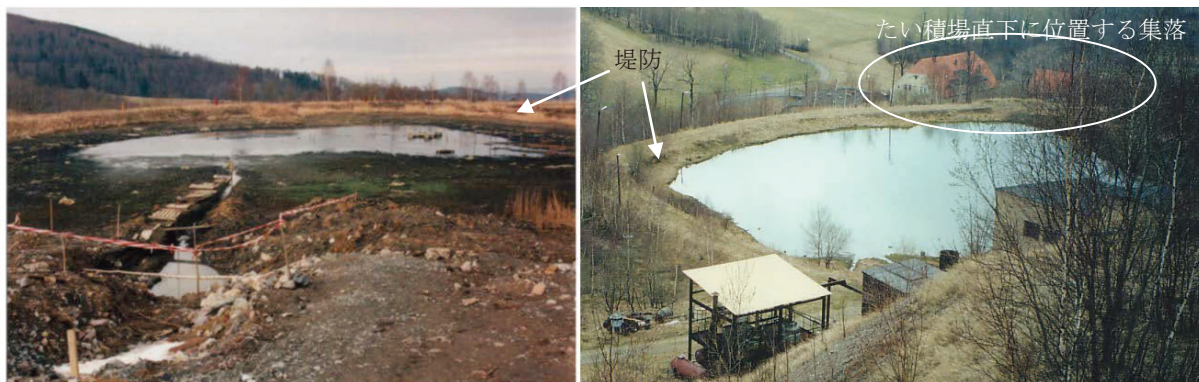
Fig. 1 Situation on site prior to remediation
