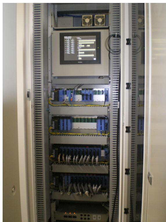
Photo 12 Inside of PPS control panel.
