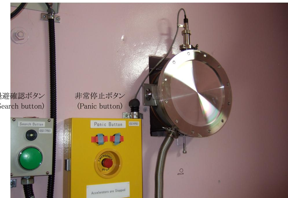
Photo 8 Panic and search buttons in neutron instrument room No.10.
