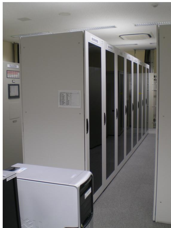
Photo 11 PPS control unit in MLF control room.
