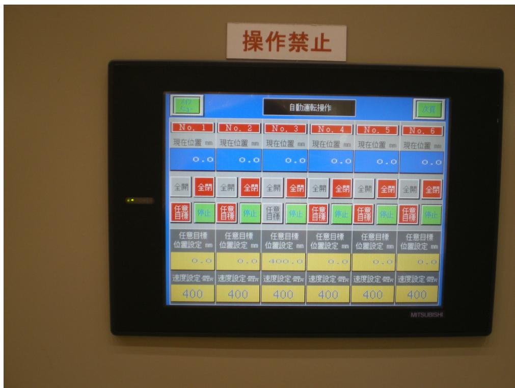
Photo 6 Display/Operation panel on shutter local control board.
