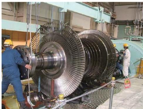
Photo 3-5 Inspection of turbine
