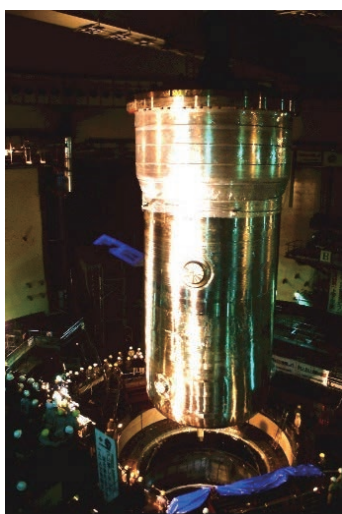
Installation of reactor vessel
