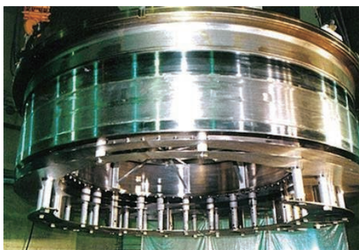
Photo 7-3 Installation of shield plug
