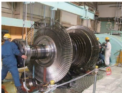
Photo 3-5 Inspection of turbine
