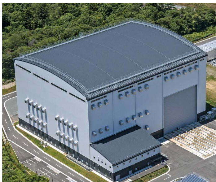
Figure 3.1.1 A Photo of the Full-scale Mock-up Building as Used Area of Transceiver Testing
