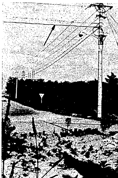
Fig. 47 Coaxial cable on the pole
