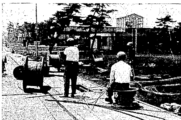
Fig. 46 Coaxial cable in pit
