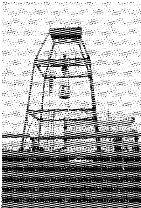
Photo.11 Tower used for free drop tests
