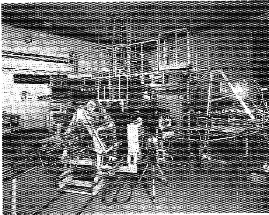
Fig.1 Photograph of the JAERI AVF cyclotron.
