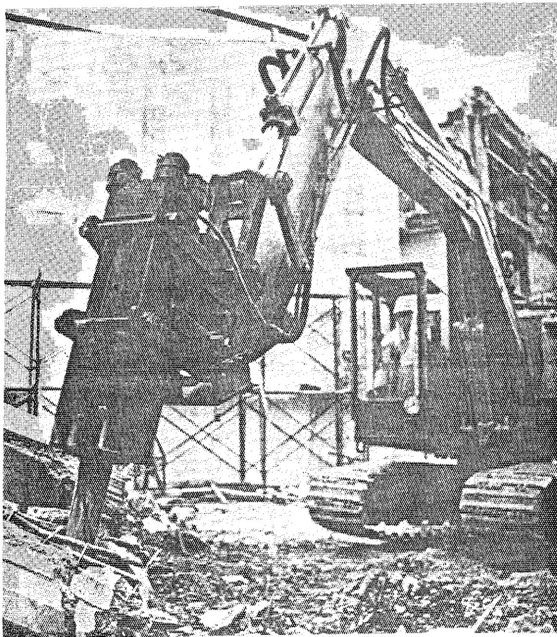
Photo 2.2.3 Demolition by a Giant Breaker 10)
