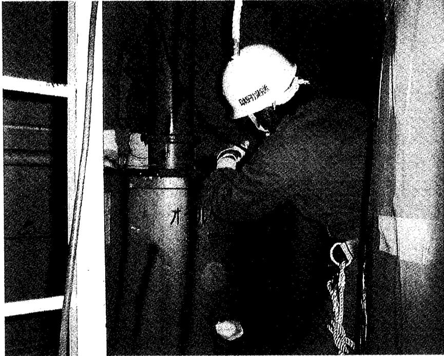
Fig.4.52 Dismantling of Oil Dumper
