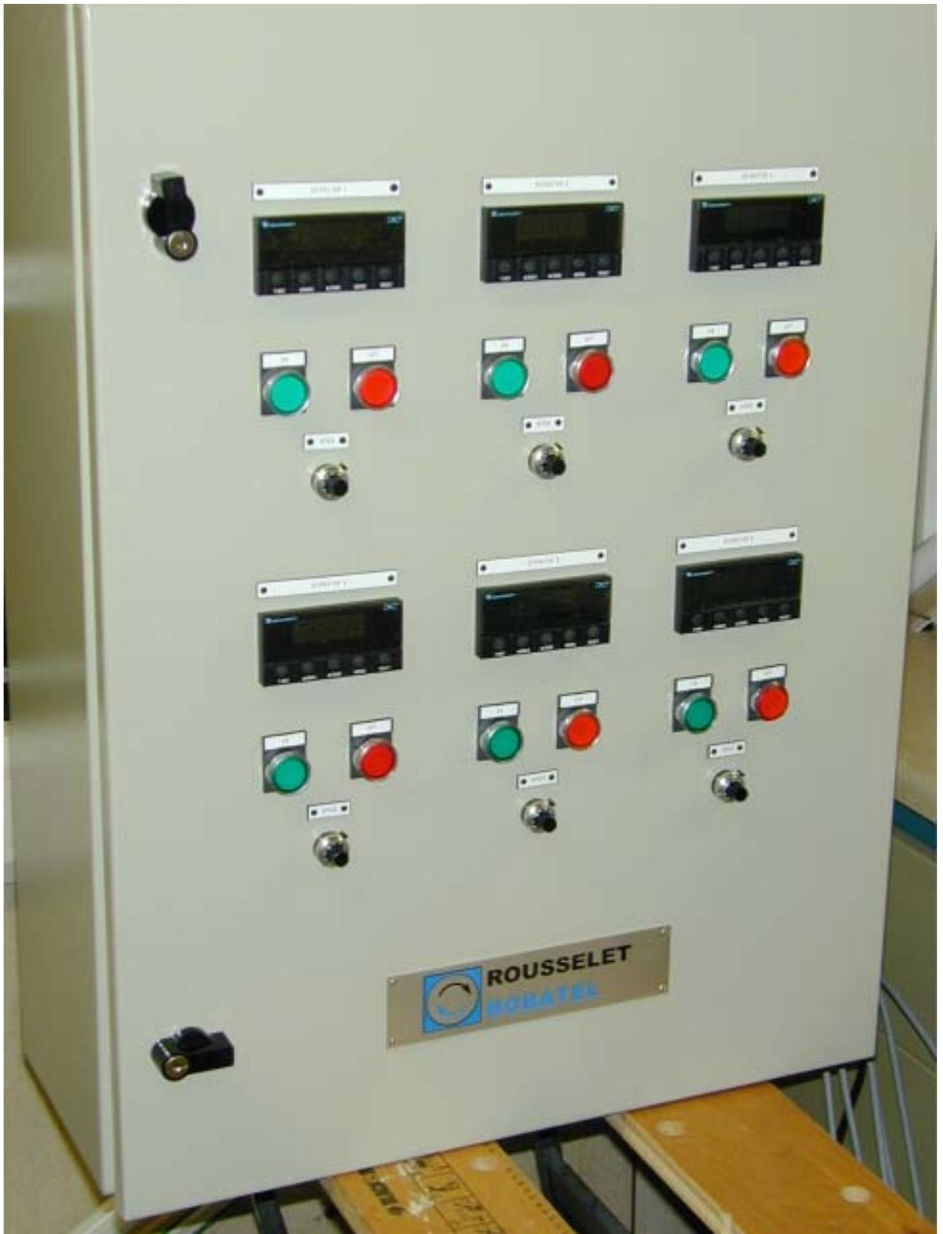
**Photograph 7. Control panel for Rousselet/Robatel BXP012 contactors**
