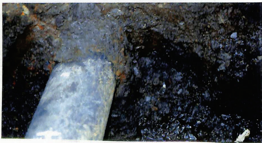
photo 1 Condition of Soil Around Pipe (Hazawa)
