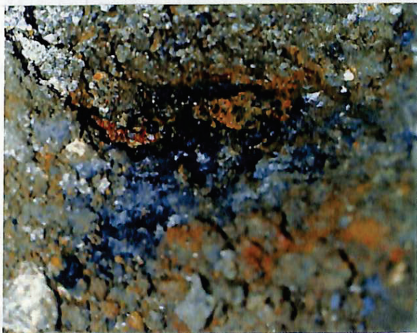
photo 2 Condition of Soil Around Pipe (Hanasaki)
