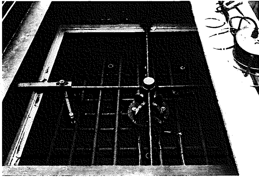
Photo. 2.2.2-1 配筋状況 Photo. 2.2.2-1 Arrangement of Reinforcing Bar
