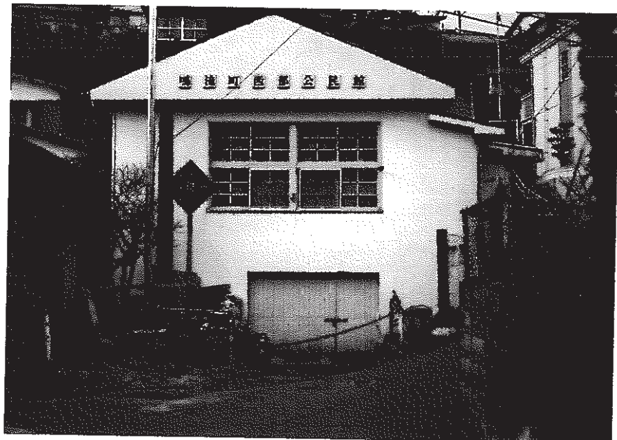
Photo 2-4 Remain of Water Service Tunnel of Narutaki Town
