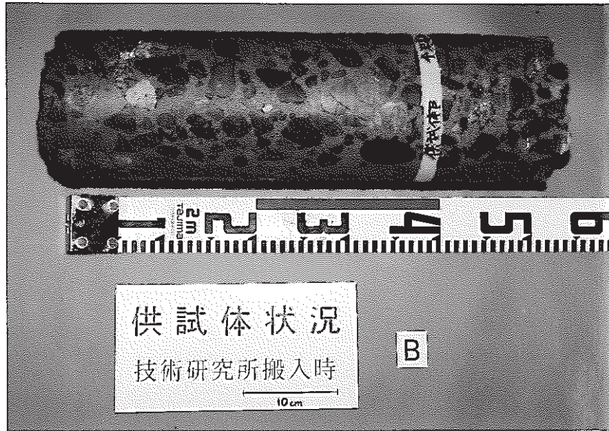
写真-15 前面部コア側面 Photo.-15 Side Surface State of Core (Riverside)
