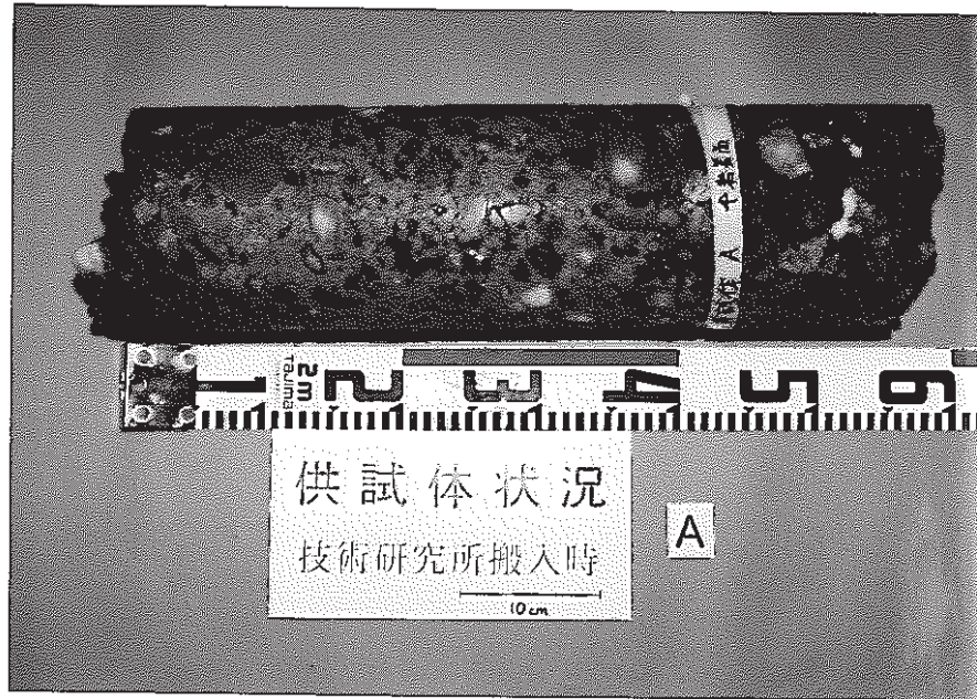
写真-13 背面下部コア側面 Photo.-13 Side Surface State of Core (Lowerpart of Landside)
