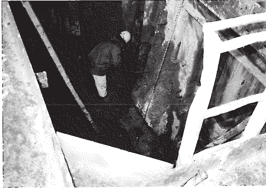
写真-8 前面部人力掘削状況 Photo.-8 Excavation at the Point of Riverside
