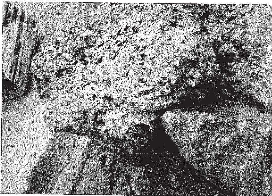
写真-4 背面下部表面状態 Photo.-4 Surface State of Concrete (Lowerpart of Landside)
