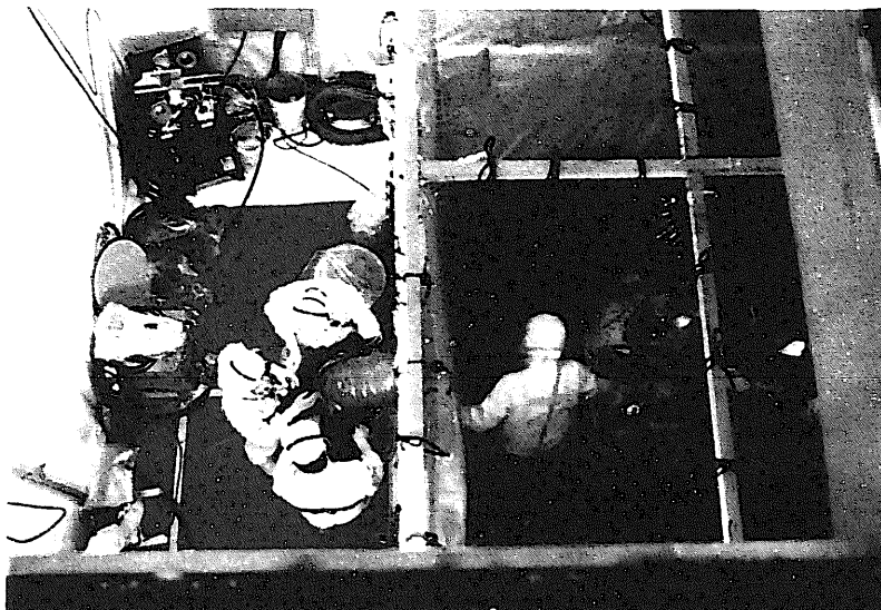
A temporary containment house
